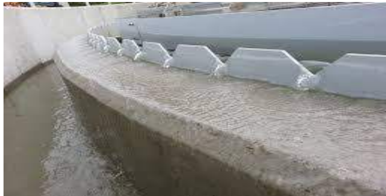
Fig.18 V-noches outlet weir
